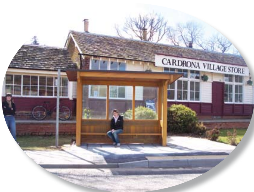
New bus shelter at Cardrona
