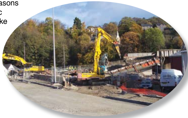
Demolition of Station Bridge in Galashiels
