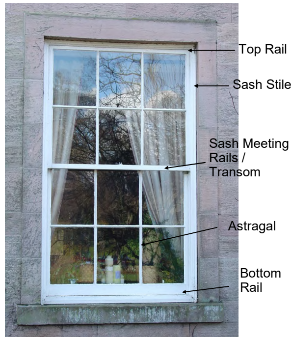
Figure 16: Traditional Window Details
