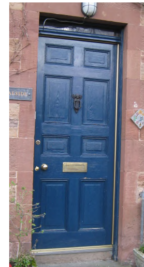
Figure 23: Example of a Panelled Main Entrance Door
