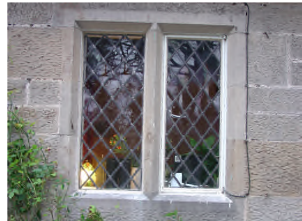
Figure 16: Traditional Metal Window with Lead Detailing on a Residential Property
