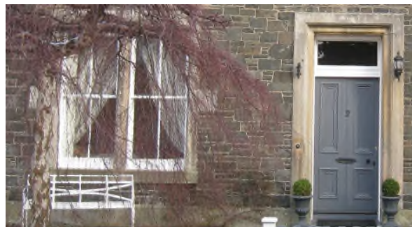
Figure 1: Historic Windows and Door - Peebles
