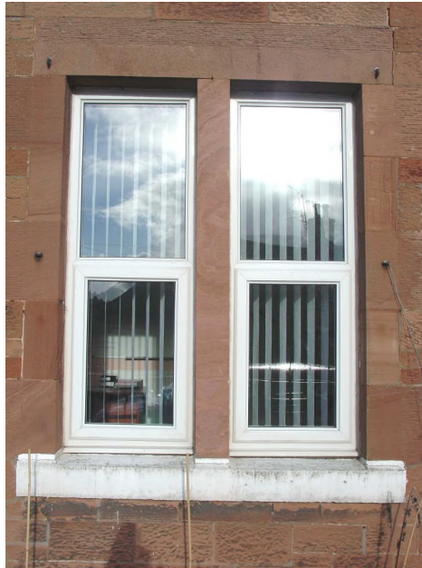
Figure 19: Replacement Window within stone opening, with mid hung sash. This results in a ‘heavy’ appearance on the lower half of the window.
