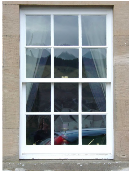
Figure 14: 6 on 6 Sash & Case Window
