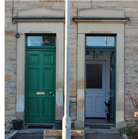
Figure 28: Matching Traditional External Doors (with internal door in entrance) - retaining matching doors on a street assists in protecting the character and appearance of the street.
