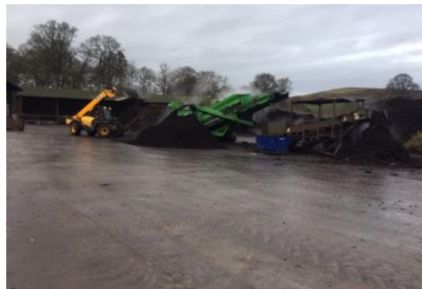
Figure 4 - Biomass processing and transfer plant
