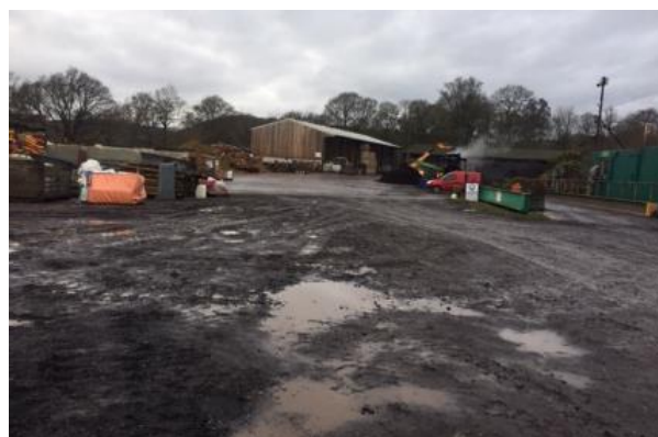
Figure 5 Biomass processing and transfer plant
