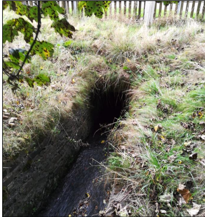
Photo 3: Cross Burn brick culvert beneath Edinburg Road (looking west)
