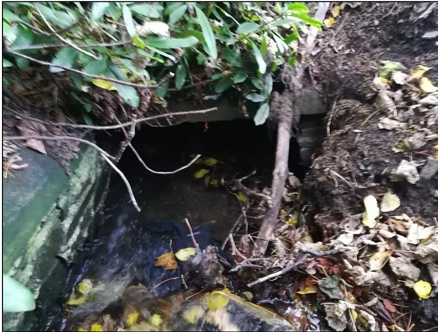
Photo 1: Cross Burn farm crossing 1 (farthest upstream)
