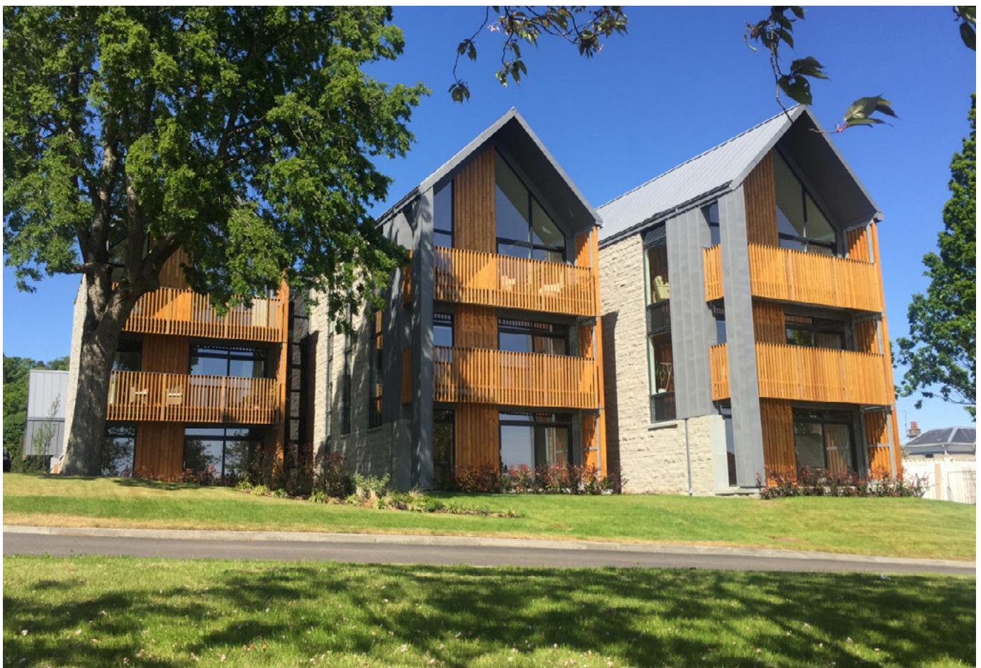
Whiteburn Projects: Parkview Phase 3, Dundee HFS Private Development of the Year Small - 2017
