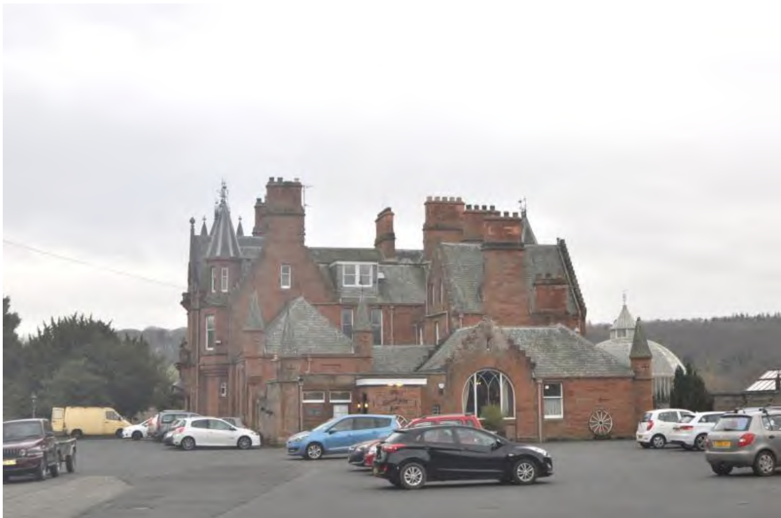
Figure 5.10 View of Kingsknowes from hotel carpark. The conservatory can be seen to the right of the house
