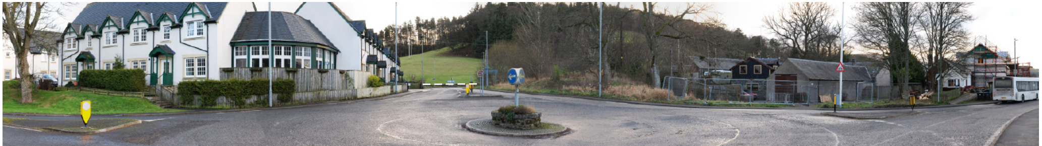
VP5 - Roundabout at approach to Cardrona from the west
