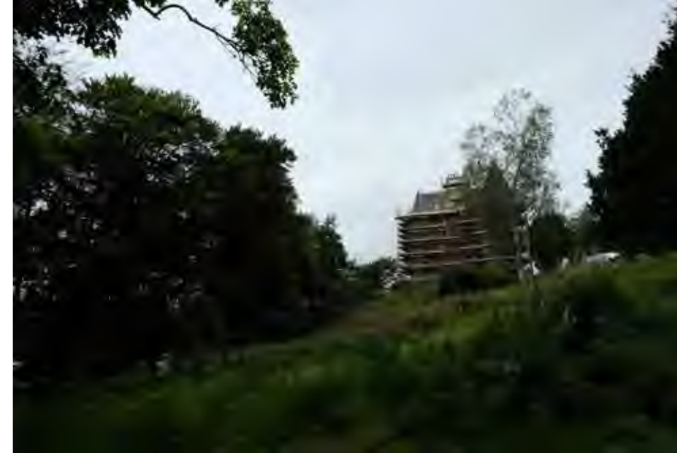
Castle Venlaw sitting above the site, currently undergoing refurbishment works.
