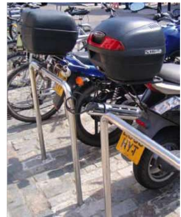
Note: cobbles are not appropriate surface treatment for PTW parking
