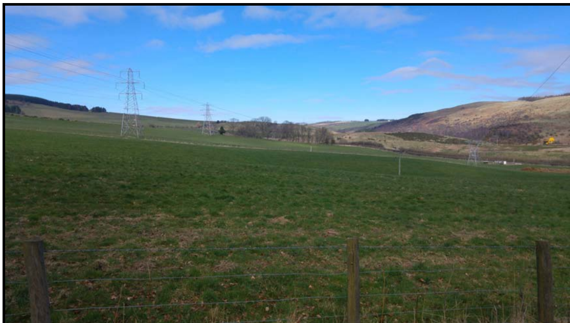
Figure 3: View across site showing two main overhead power lines and gas pipe markers
