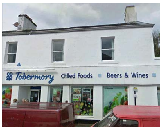
A food store on the Tobermory harbour frontage serves both the town and visiting leisure craft
