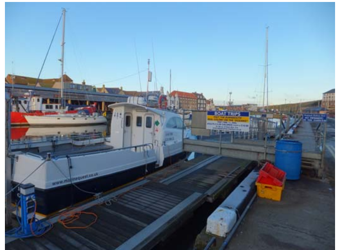
The pontoon on the Middle Pier
