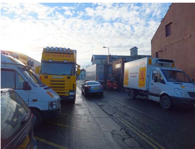
The needs of large scale transport now dominate Harbour Road, and the quayside can often take on the character of a marshalling yard for the adjacent commercial premises.
