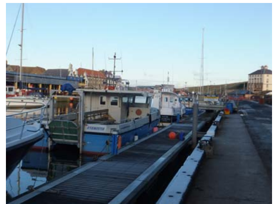
Floating pontoon moorings on the middle pier
