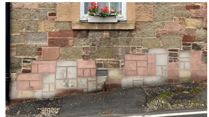
Figs. 53 and 54: over-scaled non-traditional dormer, and poor quality repairs to stone
