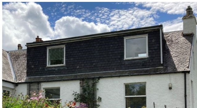
Figs. 53 and 54: over-scaled non-traditional dormer, and poor quality repairs to stone
