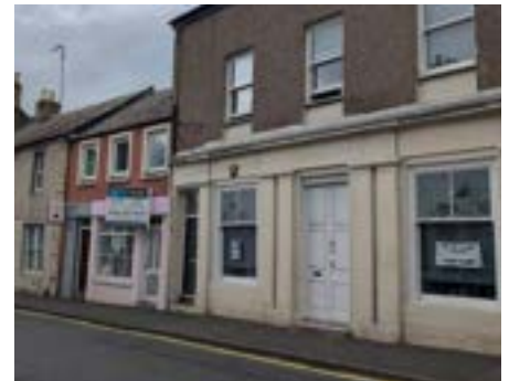
Existing vacant units
