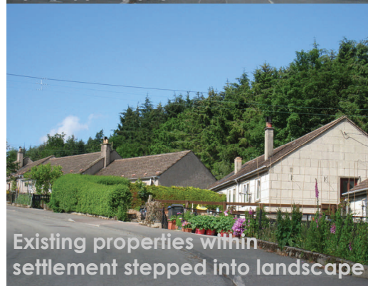
Old stage Road facing south east towards the site
