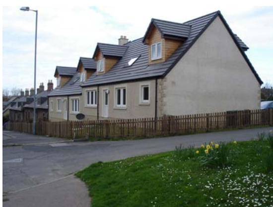
Fig. 11: Parking accessed around back of property
