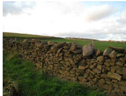
Figure 6 - Dry Stone Boundary Wall of site
