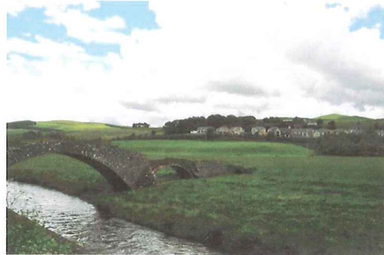
Existing view from old bridge on A7
