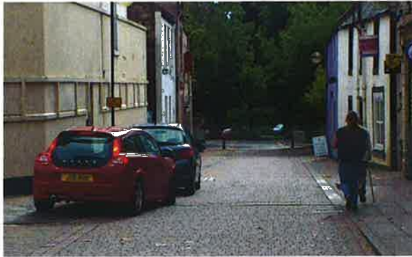
Photograph of Baillie's Entry: note the relatively narrow carriageway width and the shared surface, with no change in level between the carriageway and the adjoining footways.
