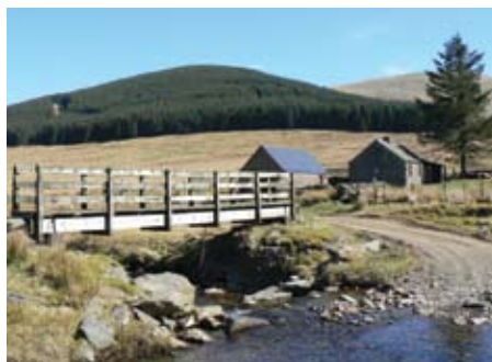
Ettrick Pen behind Overphawhope Bothy
