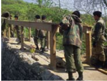
Abbey St. Bathans bridge, Gurka rebuilt
