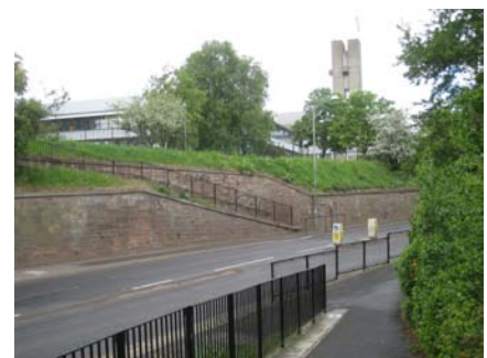
Two ramps to overcome the grade separation at the main road
