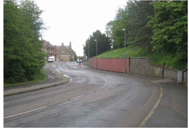
The main road where the railway bridge used to be. Its retaining walls and embankments, now partly shrouded in mature screen planting, present a formidable physical barrier which splits the village east from west.
