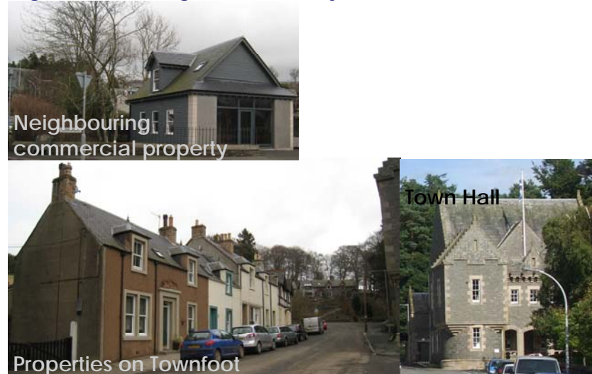
Figure 4 - Buildings in the Vicinity
