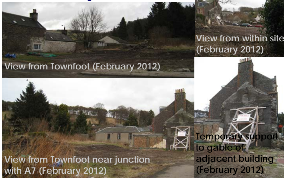
Figure 3 - Site following Demolition of Buildings
