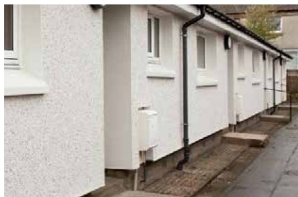
After external wall insulation
