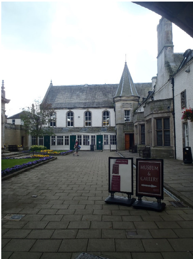
Courtyard – showing signage pointing to principal stair access for the building and showing the War Memorial (just seen to left), entrance to Registry Office / Burgh Chamber and Burgh Hall
