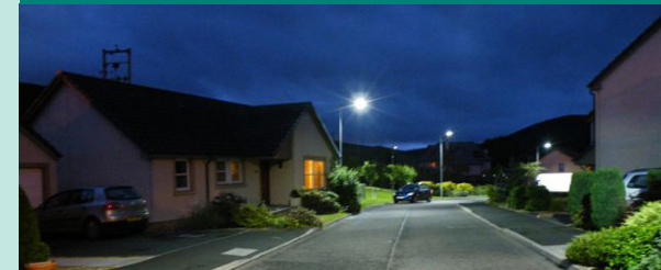
New LED Lighting
