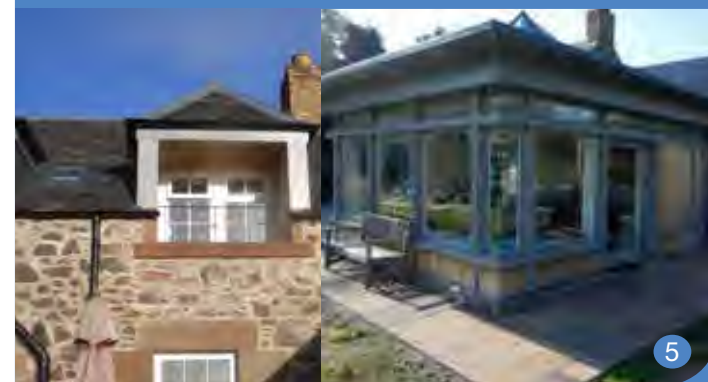
Existing Buildings - Steward's House, Frogden
