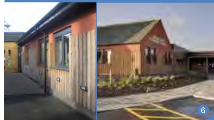
Existing Buildings - Newlands Centre, Romanno Bridge
