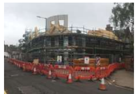
New Town Centre Development
