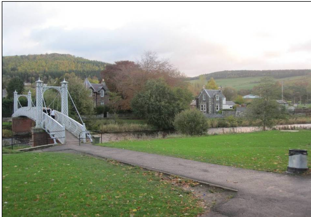
Figure 4.2 Existing footbridge and proposed location of crossing B1 (to right)
