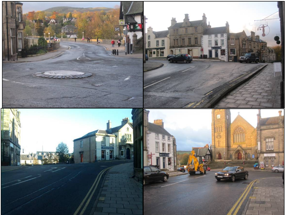
Figure 2.5 Views of roundabout to the north of Tweed Bridge
