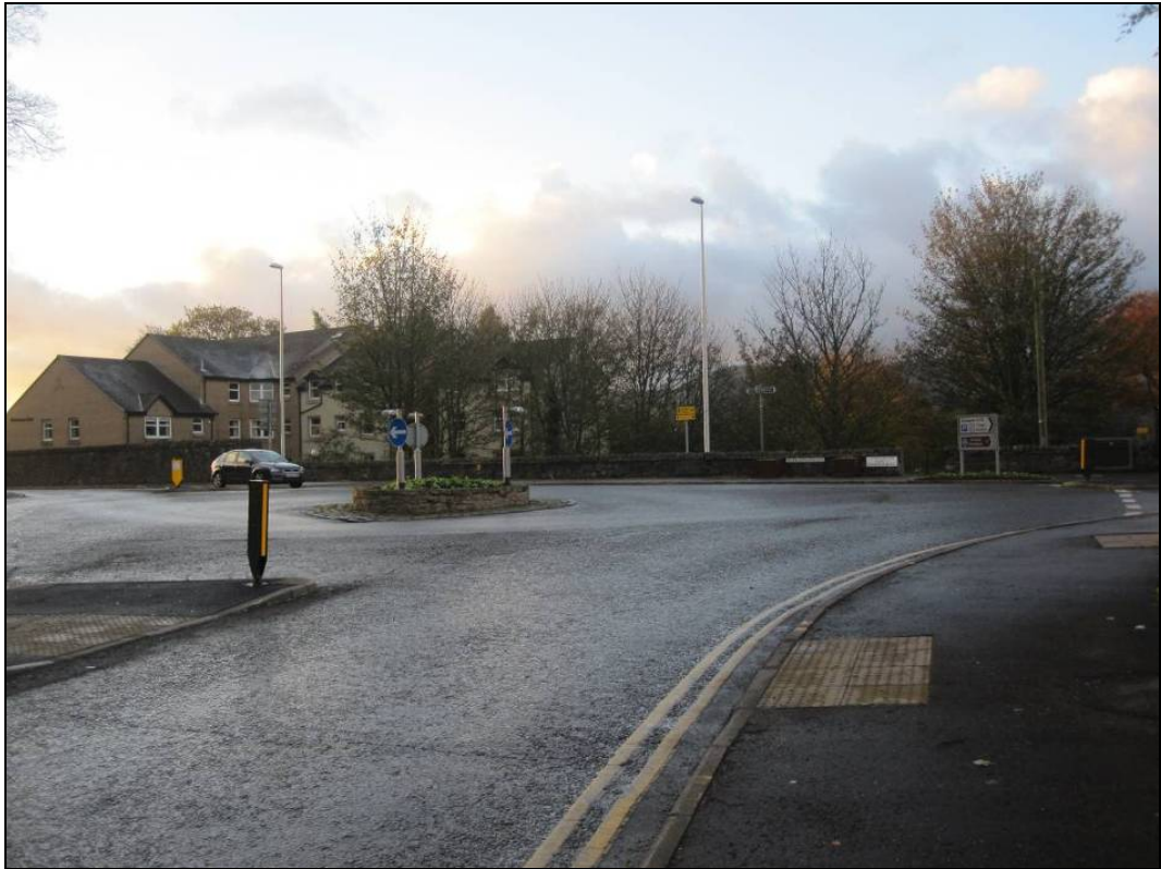
Figure 4.3 Existing A72 / A703 roundabout looking south from Edinburgh Road
