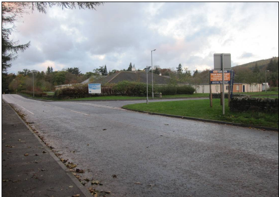
Figure 4.10 Existing entrance to Cavalry Park business park
