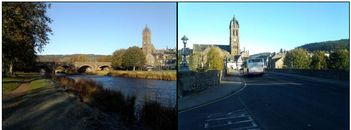
Figure 2.4 Tweed Bridge in Peebles
