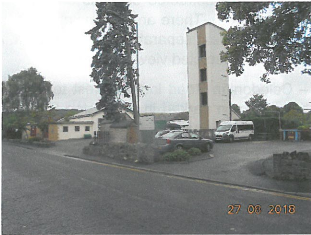
Caledonian Road – North side with Fire Station & Ambulance Station
