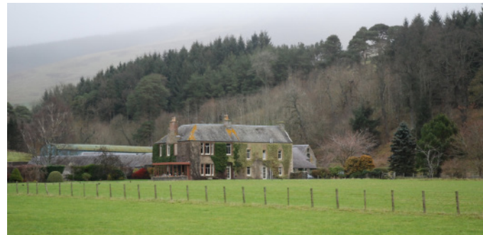
B-grade listed building at Nether Horsburgh - buildings set against a woodland backdrop
