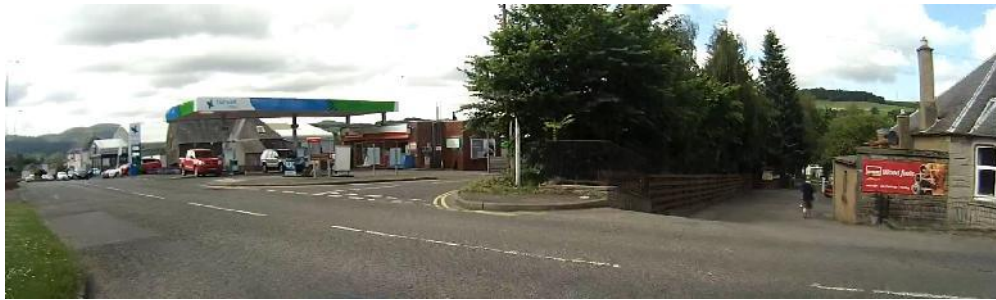
Photograph 2.9 – West side of Edinburgh Road
