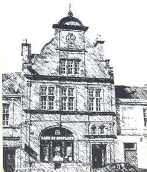
Bank of Scotland Building
