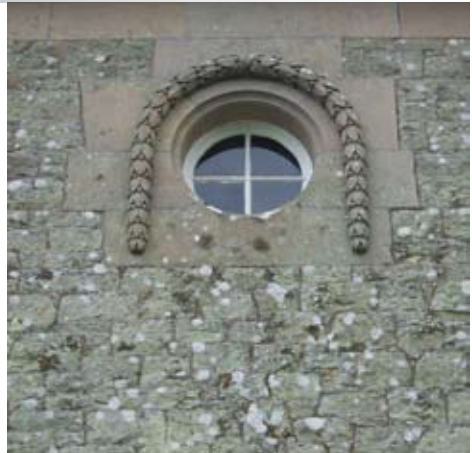
Romanesque revival detail on Manderston building
