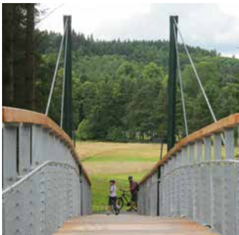
New bridge for Tweed Valley Railway Path
