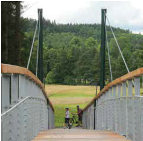
New bridge for Tweed Valley Railway Path
