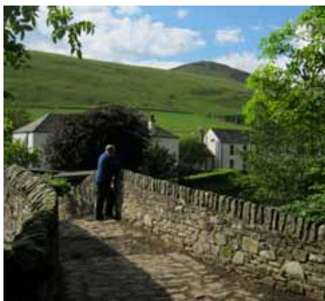
Looking at the Leithen Water on Cuddy Brig
