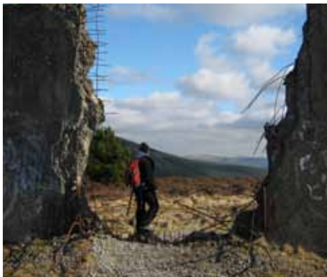
The opening into the disused water tank
