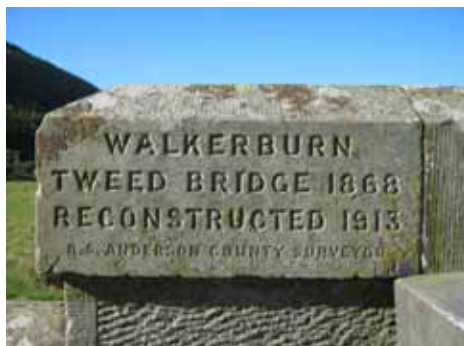
Walkerburn Tweed Bridge
