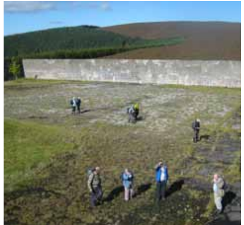
Inside the water tank
