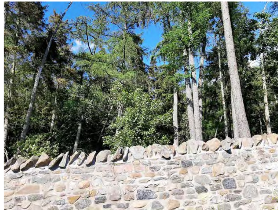
Areas of plantation forest are at the end of their lifespan and should be cleared for forestry management reasons. This provides future development opportunities.
