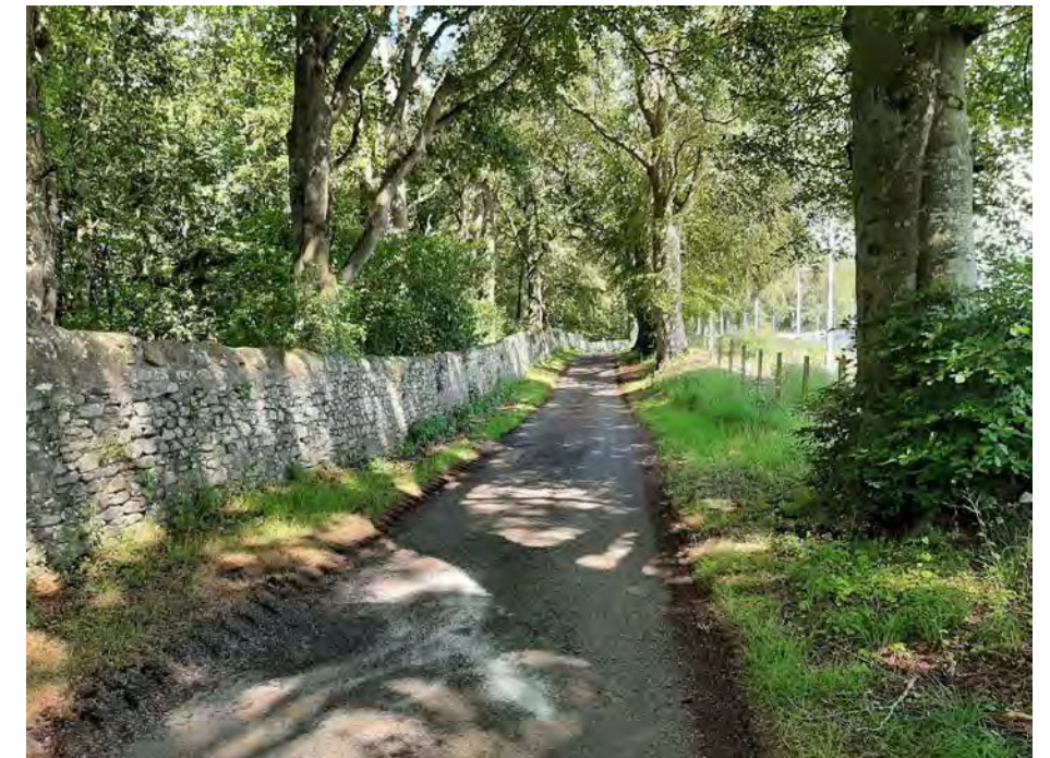
The perimeter access road with its historic wall and mature avenues should be retained and protected. This can form a new active travel corridor for pedestrian and cycle use.
