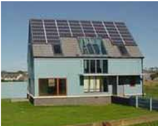
House at Ayton utilising solar energy
