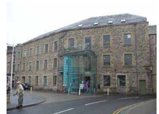
Tower Mill, Hawick, existing settlement
