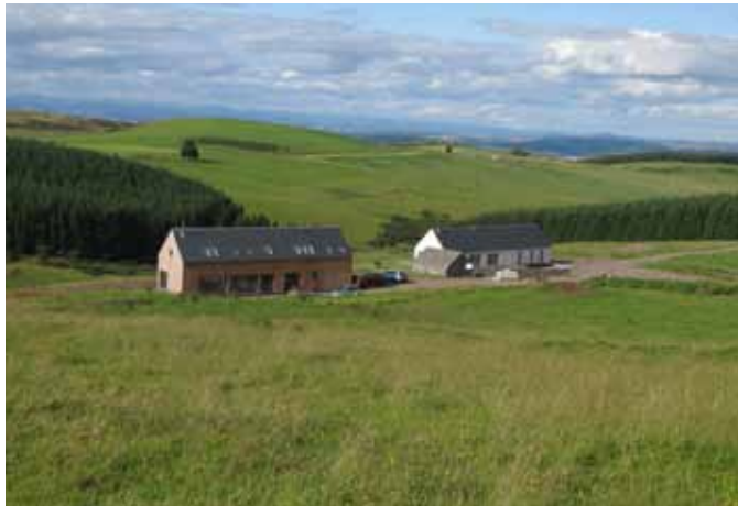
Traditional forms and materials using contemporary detailing sit naturally within the rural landscape: note the use of roofspace
