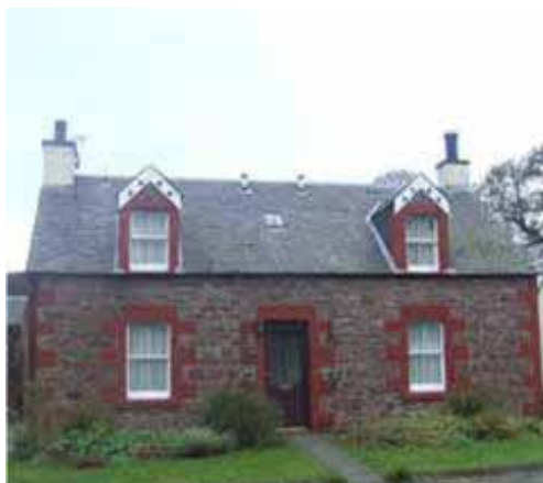
Traditional slate roof
