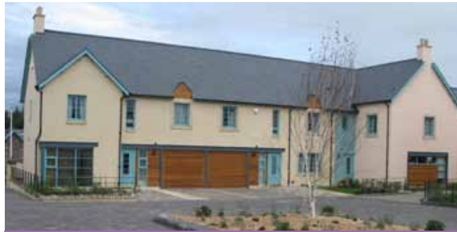
Traditional forms shaping a permeable courtyard, Lauder
