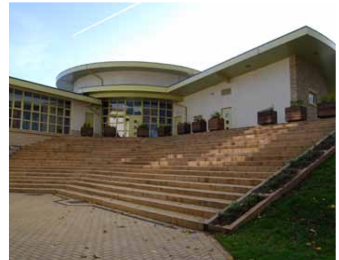
Recently built Denholm Primary School, following sustainable design principles.
