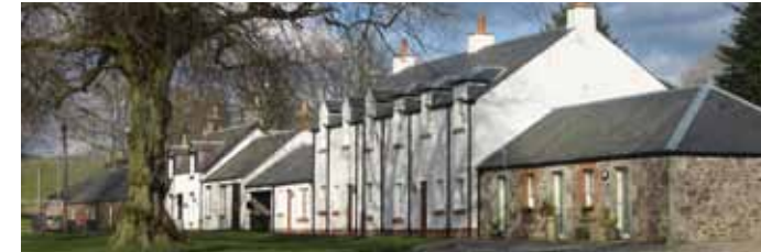
New infill can successfully contrast and complement adjacent buildings, using a similar rhythm of windows and roofline
