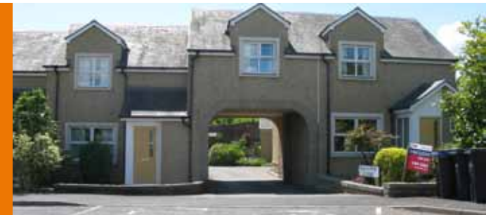
Courtyard parking with pend access at Darnick
