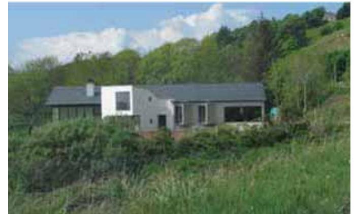
Building form working with the site features and landscape backdrop, Oban
