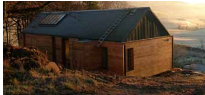
House at Heriot using well established tree shelter
