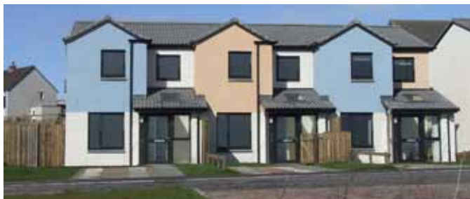
Coherent building forms, working with the microclimate and each other to optimise solar gain and shape space (Bain Swan Architects)
