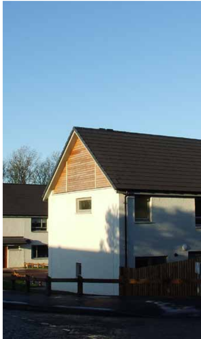
Appropriate roof pitch applied to recent housing in Kelso, also using well-proportioned gable windows to provide overlooking (Smith Scott Mullan Architexts)
