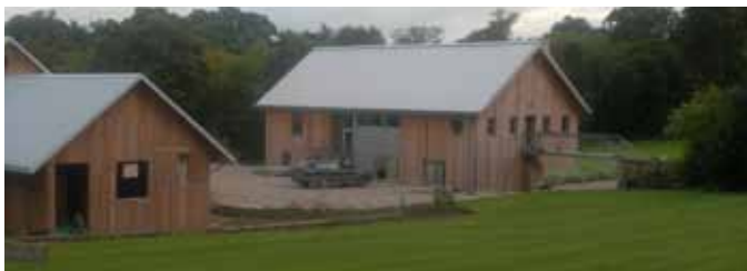
In an established landscape setting, an opportunity to explore innovative forms materials presents itself
