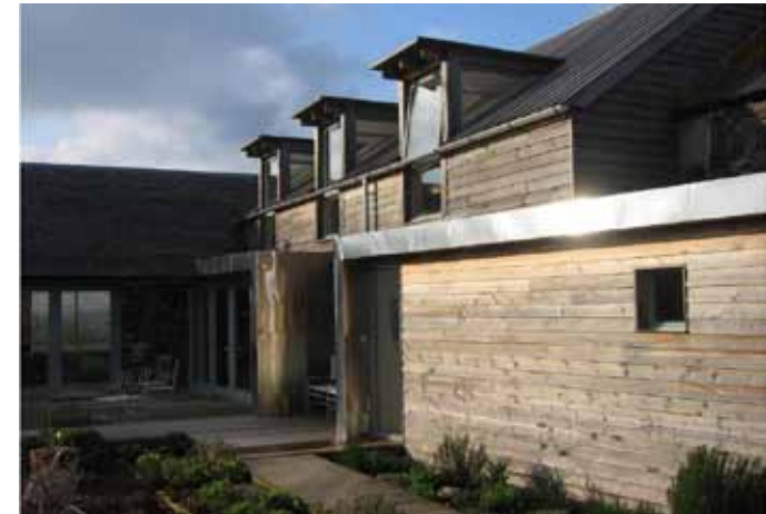
Working in harmony: windows, roofline and wall elements combine to create an innovative response with strong traditional references
