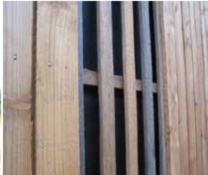
Figure 2 : 150 x 22mm on 60 x 22mm dressed front face only, with 10mm gap on front face, untreated
