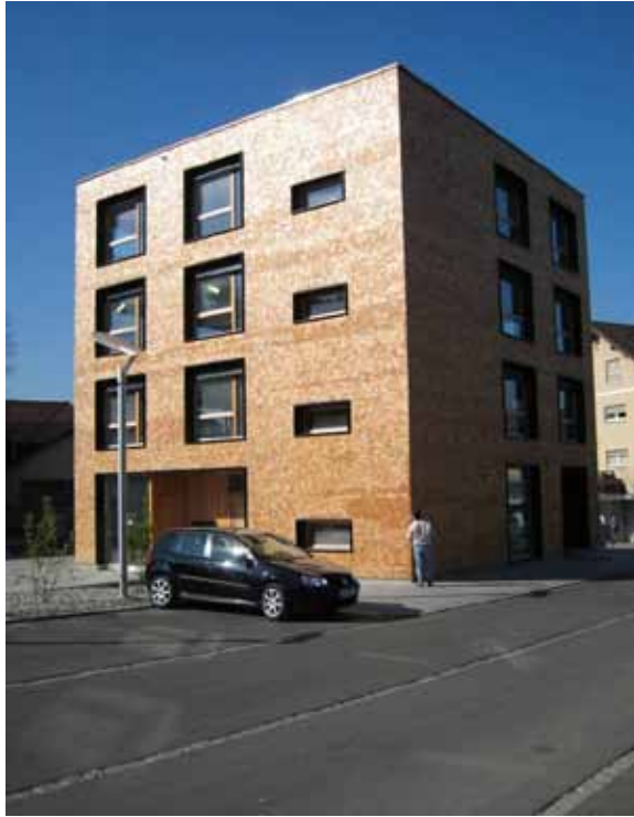
Figure 15 : Larch shingles on all four elevations of a four story office in Vorarlberg, Austria.
