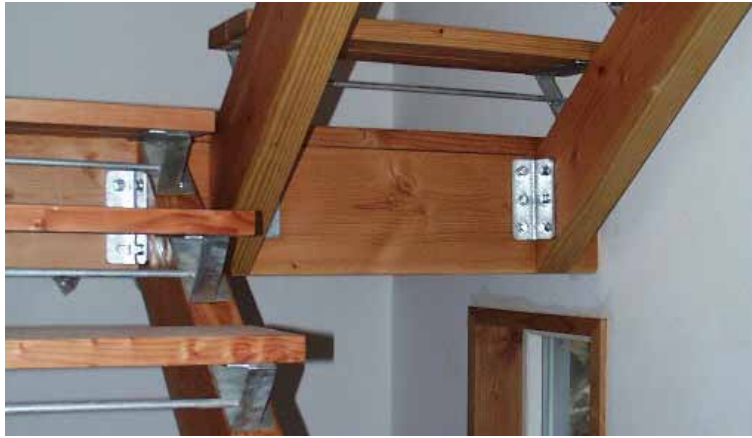
A staircase in Scottish Douglas fir and steel in a contemporary design by North Woods Construction Ltd. Photo: Bernard Planterose
