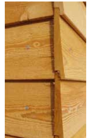
Figures 7 & 8 : 150mm ship lapped (feathered) boards, with a face of 135mm, off saw, untreated.
