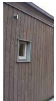
Figure 4 : 150 x 18 on 60 x 18mm with 9mm gap on front face, dressed three sides and stained
