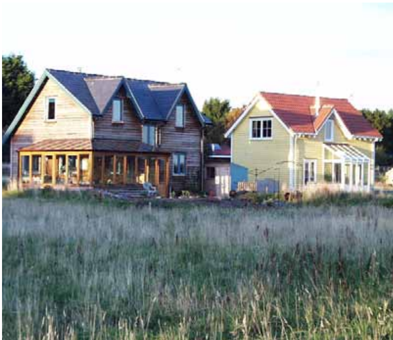
Contrasting approaches to timber treatment seen at Findhorn Eco-village. The house on the left is being left to weather naturally whilst its neighbour takes a 'retro' Scandinavian approach with brightly coloured, opaque paint to all exposed timber. Photo: Bernard Planterose
