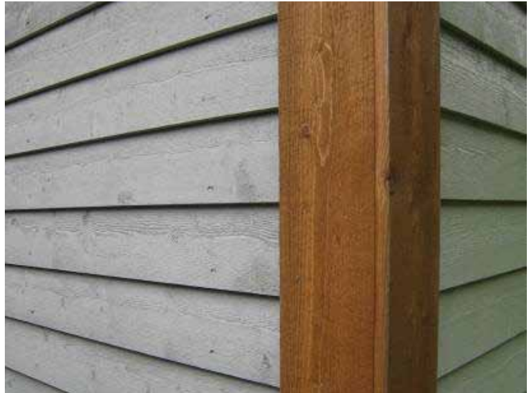
Figure 6 : 150mm feather edged boards, with a face of 135mm, off saw, painted.
