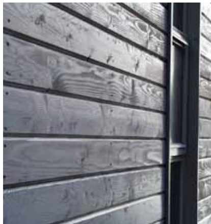
Figure 11 : 125mm finished face, 20mm deep, fully profiled and dressed boards, stained.
