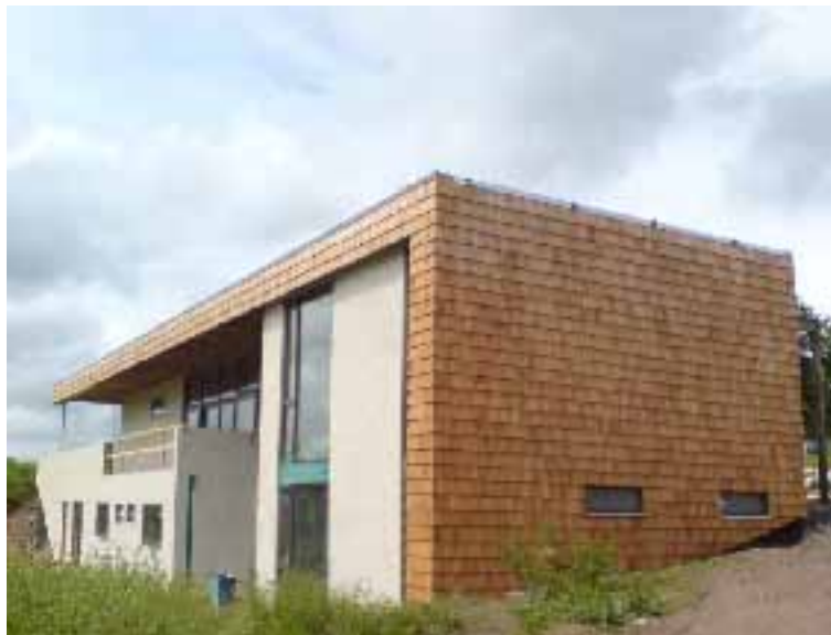
Larch shingles in combination with white render on a contemporary house in Midlothian. Architect: Icosis. Photo: Icosis
