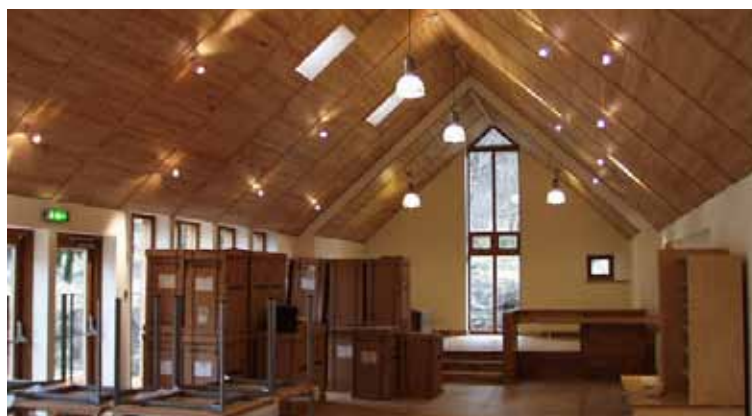
The ceiling of the Glencoe Visitor centre utilizes home-grown birch in an un-nailed system. Photo: Bernard Planterose
