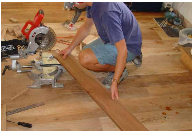
Floor of home grown elm, sourced and machined in the Borders by Abbey Timber. Photo: Willie Dobie
