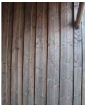
Figure 1 : 150 x 18mm on 150 x 18mm with 100mm gap on front face, off saw, untreated.
