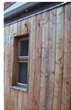
Figure 3 : 150 x 20 on 60 x 20mm with 10mm gap on front face, off saw untreated
