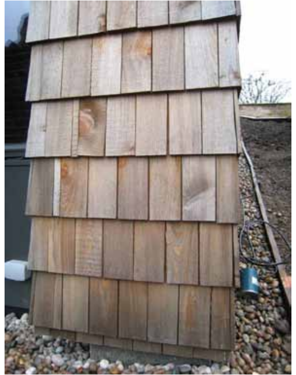
Figure 16 : Larch shingles on parts of two elevations of house in Midlothian by Icosis.
