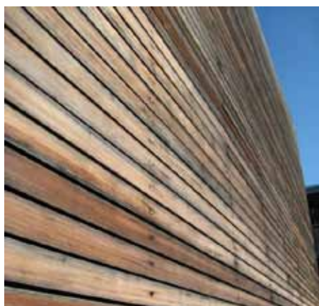
Figure 13 : 60mm finished face, 40mm deep, trapezoidal profiled boards with 10mm gaps.
