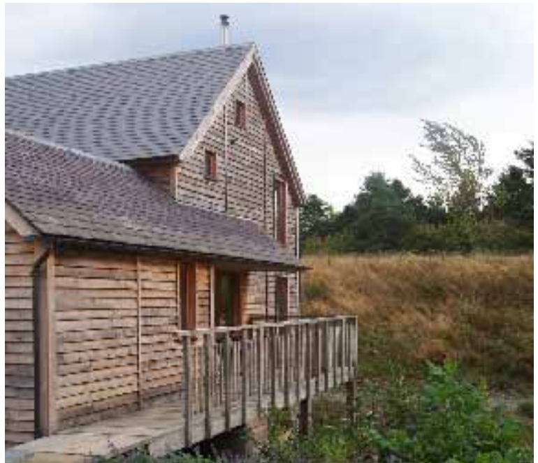
Untreated home-grown European larch turning silver on house in Borders. Architect: Sally Ruel. Photo: Sally Ruel
