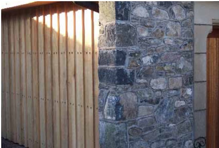
Untreated oak cladding in combination with local field stone on a house in the Borders. Architect: Sally Ruel. Photo: Sally Ruel
