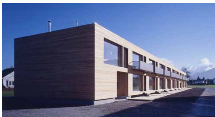
It is likely that different models of high density and lower cost housing will need to be explored. We may have something to learn from highly energy efficient central European examples such as this from Dornbirn in Austria. Architect: Johannes Kaufmann Architektur
