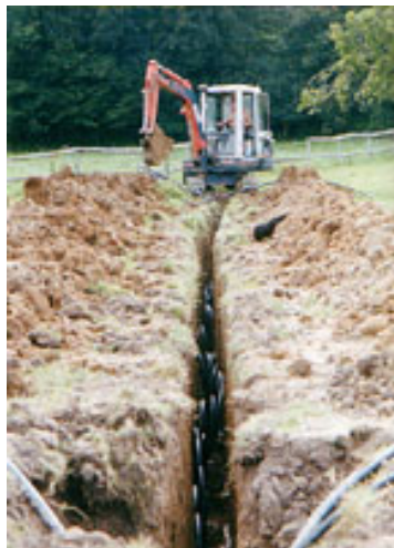
Digging the trench
