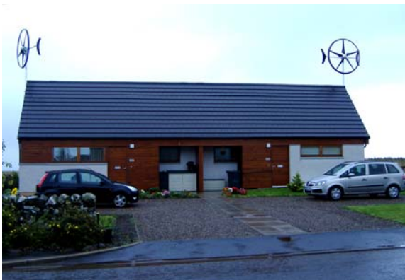
(a) Gable Mounted Micro-Turbines Whitsome, Berwickshire
