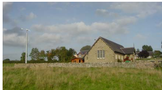
(b) Tower Mounted Wind Turbine Nenthorn, Cheviot
